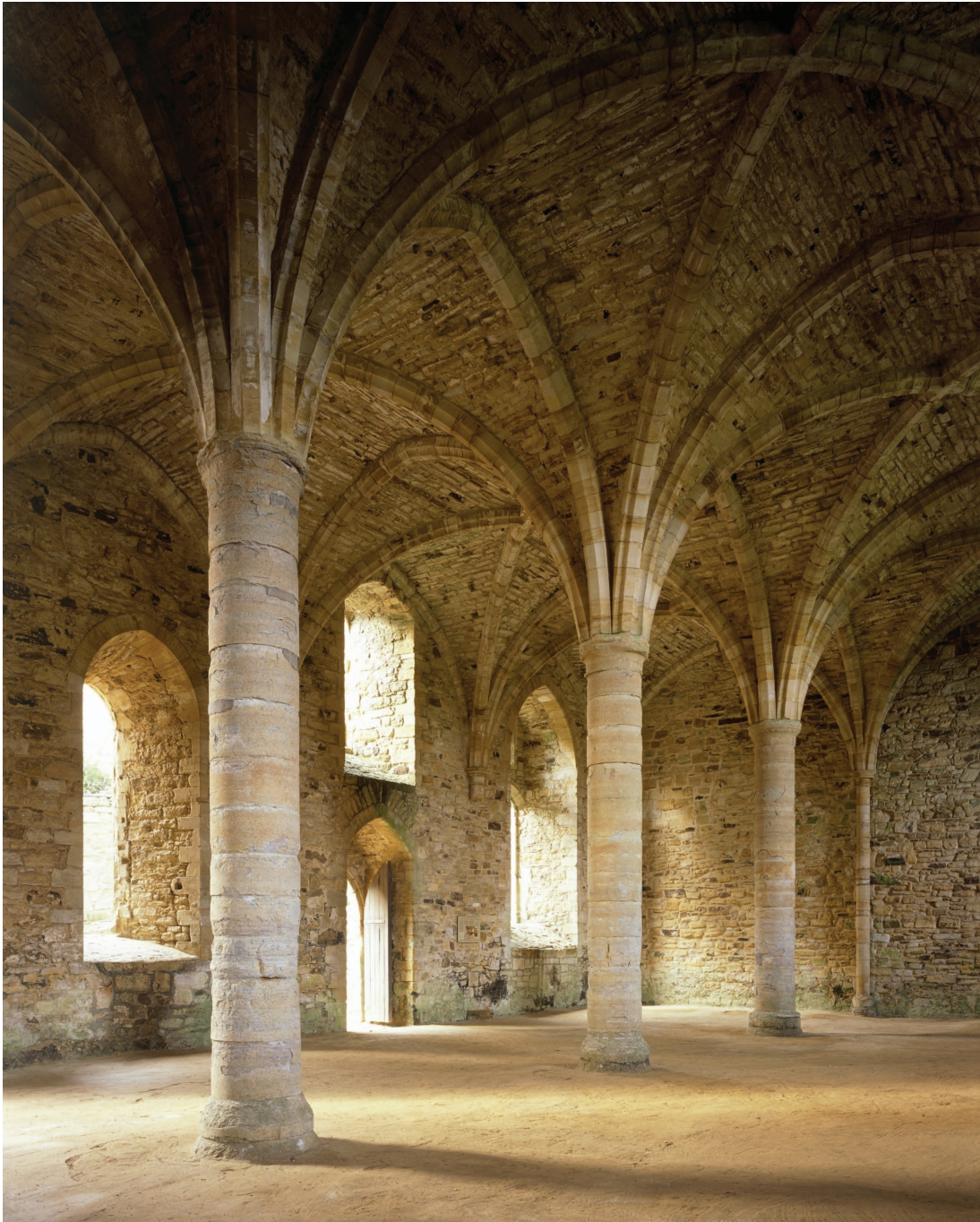
Fig. 5. The southern undercroft of the dorter range at Battle Abbey. The soaring dimensions of the space are the result of the building having to overcome the difficulties of a hillside location.
